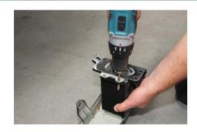
5. Bolt support to frame with M6 bolts and nuts supplied.
